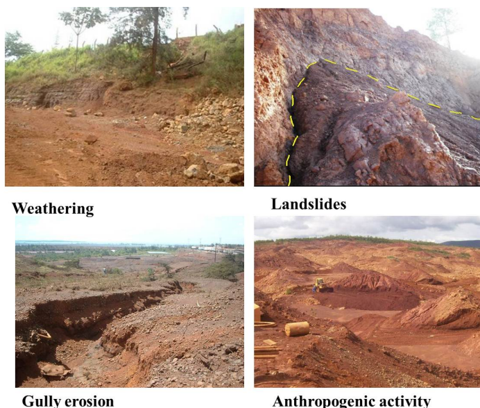
Figure 1 – External geodynamic processes and phenomena generated in the weathering crusts of Moa
