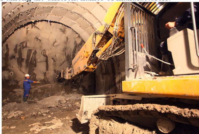
Figure 1. Tunnel drifting with hydraulic breaker on an excavator
